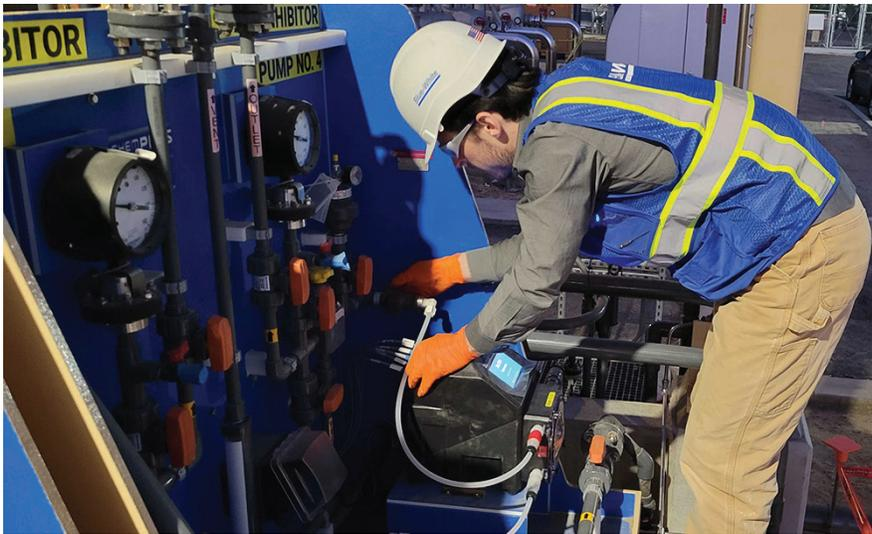
Figure 1. Chemical Feed Pumps at the Los Angeles County Sanitation District dosing sodium hypochlorite for water remediation
